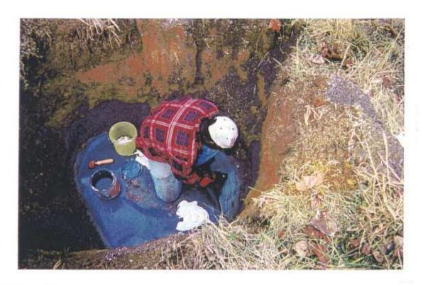
INSTALLATION OF 30 MIL PVC PATCH AND APPLICATION OF ADHESIVE (ABOVE) APPLICATION OF PRESSURE TO ENSURE STRONG BOND (BELOW)
