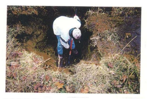
HAND EXCAVATION OF SOIL CAP NEAR MEMBRANE INTERFACE (ABOVE) EXCAVATED REPAIR AREA PRIOR TO PATCHING (BELOW)
