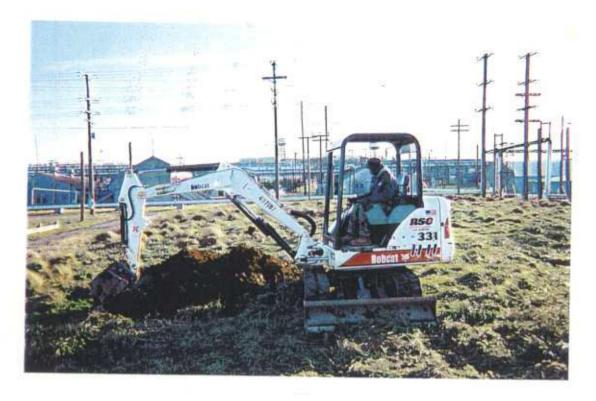
EXCAVATION OF SOIL CAP AT REPAIR LOCATON (ABOVE) EXCAVATION OF SOIL CAP AT REPAIR LOCATION (BELOW)
