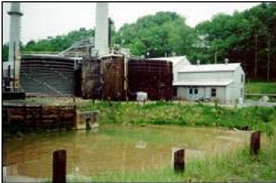
Photo 1 - Primary Settling Lagoon. Drinking water plant and boiler in background.
