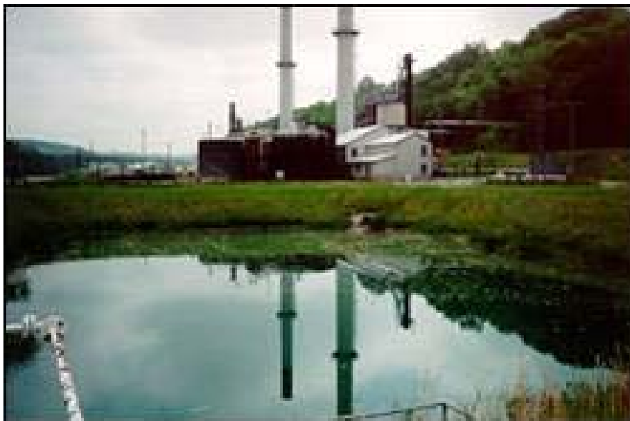
Photo 2 - Secondary Settling Lagoon (looking east).
