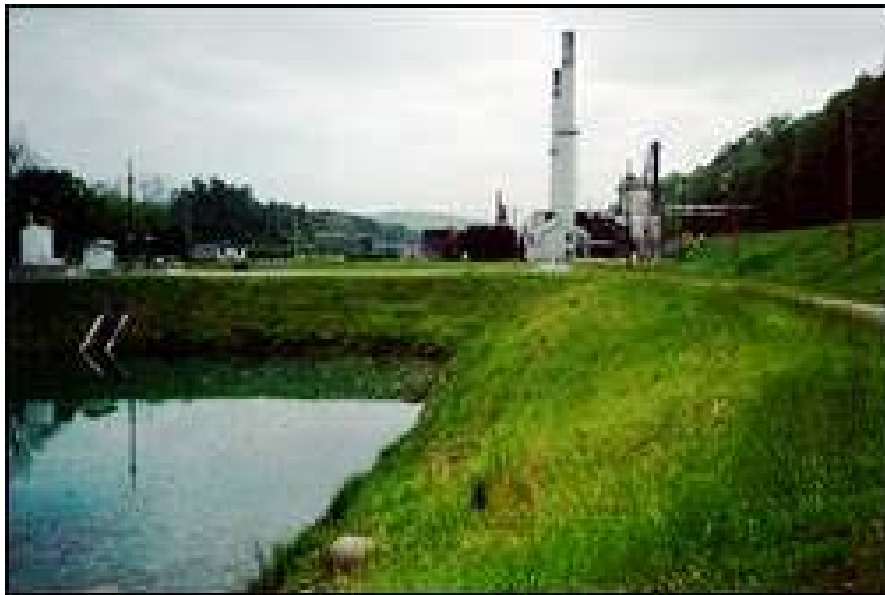
Photo 3 - Tertiary Settling Lagoon (looking east).
