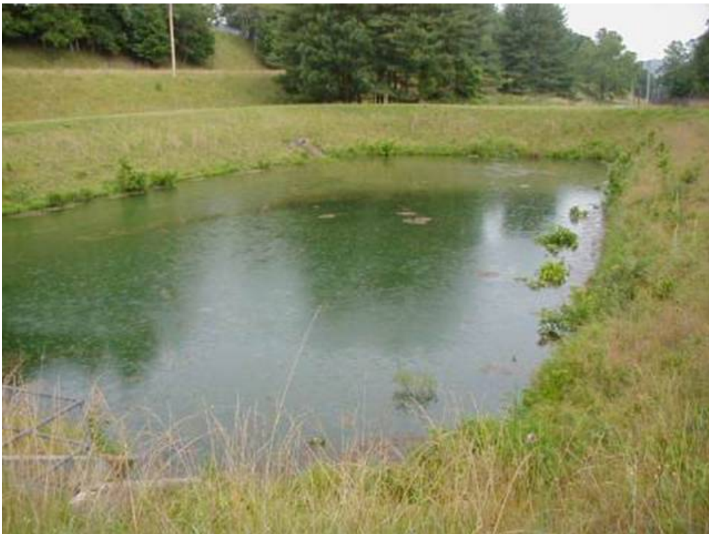
Photo 6 - Tertiary Settling Lagoon.
