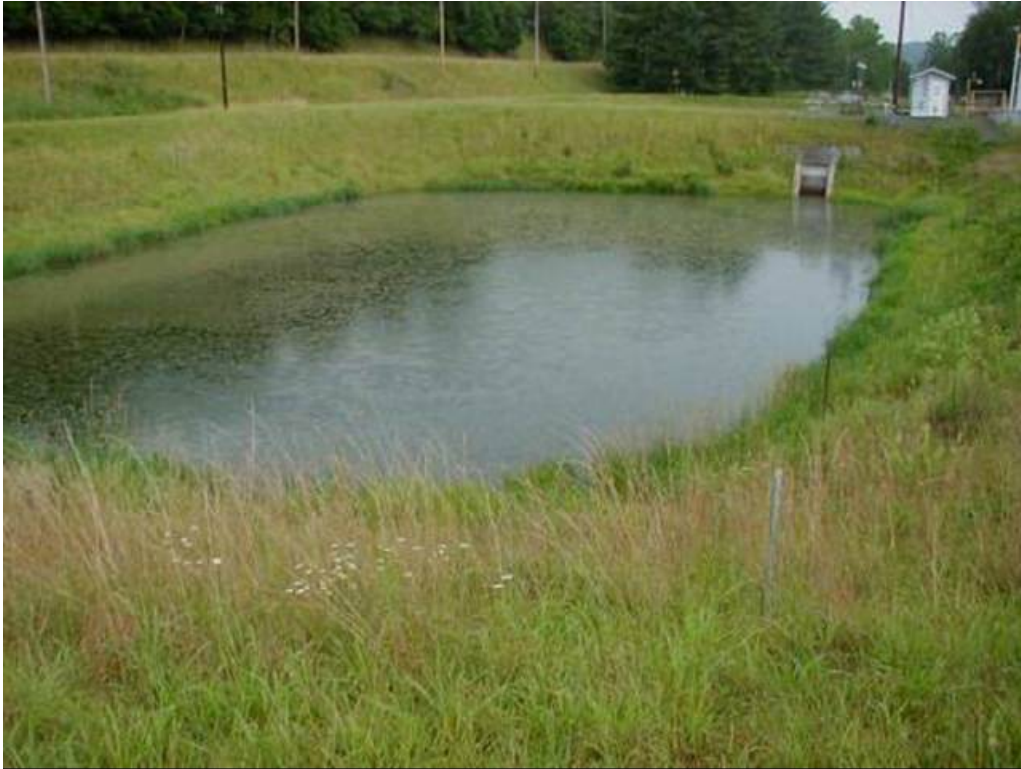
Photo 5 - Secondary Settling Lagoon.
