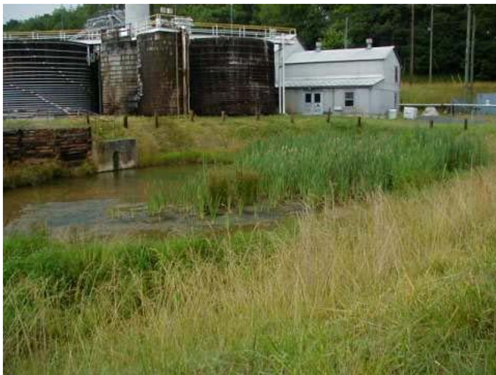
Photo 4 - Primary Settling Lagoon.
